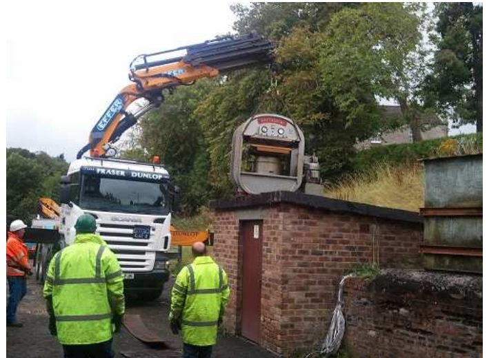
17 tonnes up and over the shed.....
