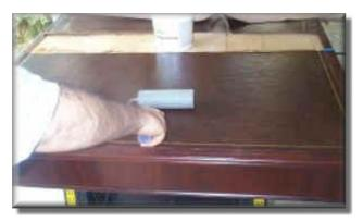
9. Now that the insert is well fitted and positioned in the centre it is time to smooth out all of the bubbles and lumps
